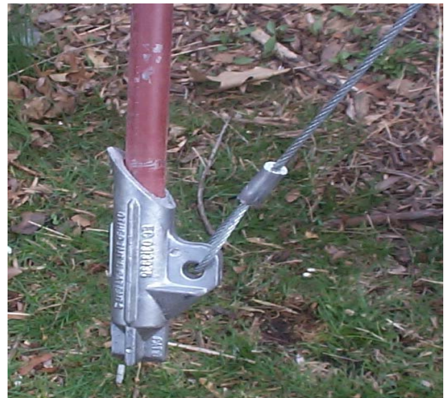
Drive Rod inserts into Anchor Head
